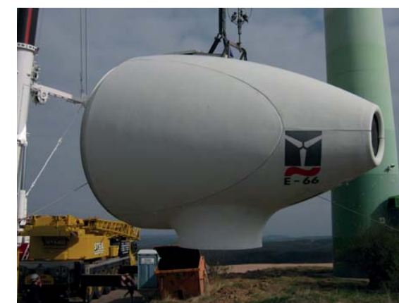
Figure 1: Retirer la salle des machines
